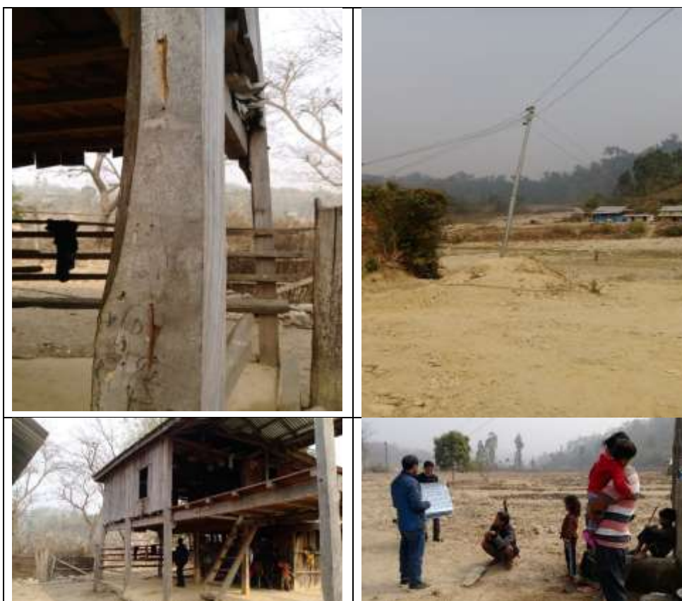
Figure 4 All pictures from Makawanpur: (Clockwise from the top left) Scar on a wooden pillar after lightning struck that left one person killed and several more injured during dinner in the evening. Local people reported that majority of lightning incidents take place on electricity lines (top right). The house of the victim family (bottom left). Lightning safety awareness on progress (bottom right)
